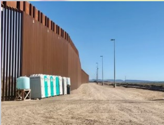
Toilets and water at the wall
